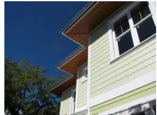
STAFF PHOTO / HAROLD BUBIL Contractor Josh Wynne built this green house in Laurel Park for a client. It will be featured on the Junior League Holiday Tour of Homes.
